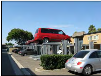
Top: Example of hydraulic parking in Europe in a garage. Bottom: Hydraulic parking in use in Santa Ana on a surface
