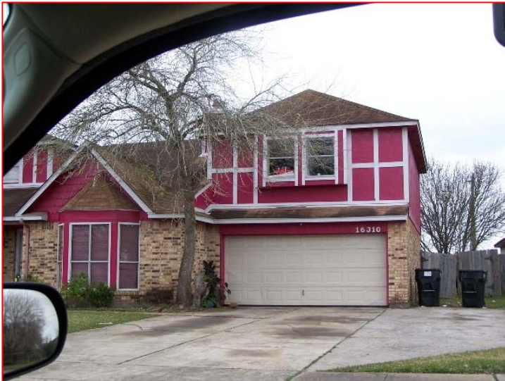
Driveway addition on right side
