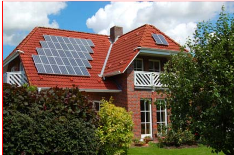
Solar panels on roof
