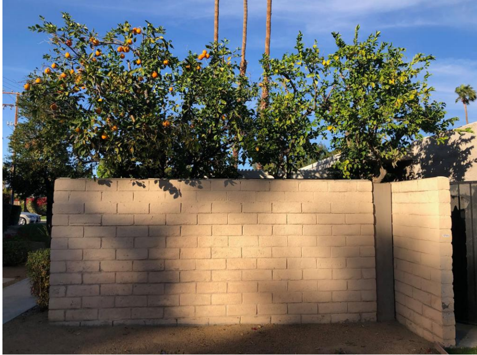
As originally drawn, most of the slumpstone patio walls, like this six-foot-high one on E. Sandalwood Drive, had slender wooden inserts at the corners. The citrus trees are inside the patio. (Photo by Claude Peck)
