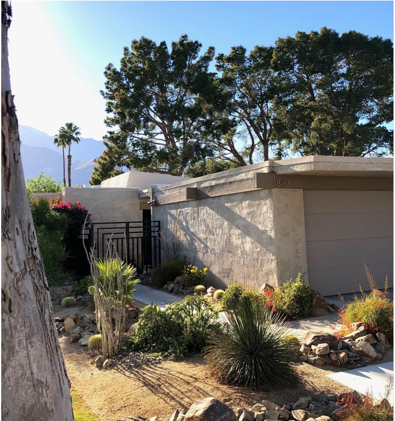
Post-and-beam construction expressed at the garage of a two-bedroom unit with recessed entry, newer gate, desert planting and rooftop HVAC enclosure. The stucco is a slightly lighter color than the Douglas fir strips.
