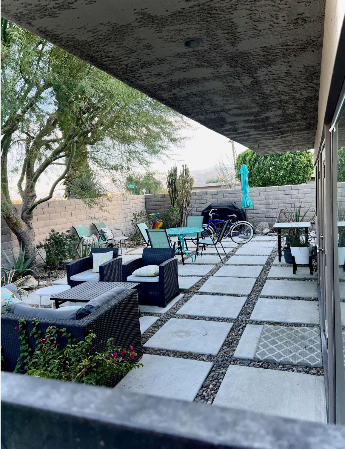
A large patio enclosed by slumpstone walls at a two-bedroom unit is typical at Sagewood, where the outdoors can be enjoyed privately or in shared pools and green spaces. Roof overhang helps shade full-height glass at right. (Photo by Claude Peck)
