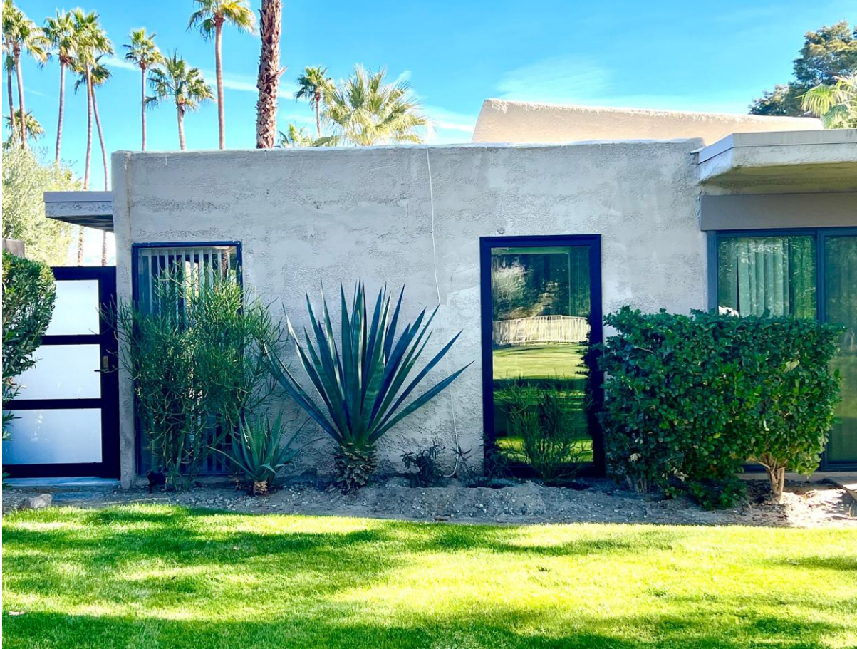
Newer gate (at left), with shade overhangs, full-height windows looking onto the park, and a slightly slanted rooftop enclosure to disguise HVAC units. (Photo by Claude Peck)
