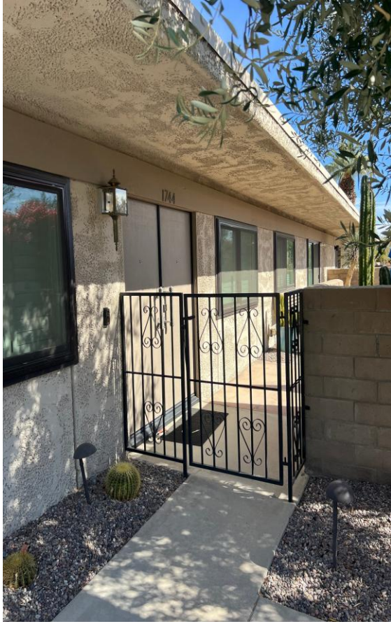
Double entry doors above, including the matching door handles, are original to some units. Current architectural guidelines advise against the scrollwork detail on the newer iron gate. (Photo by Claude Peck)
