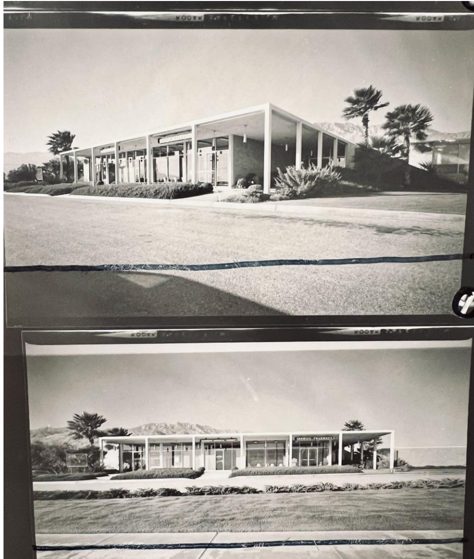
Clinics and a pharmacy were part of Wexler's gracefully porticoed 1963 Palm Springs Medical Center, across from the current-day Sagewood condos. Now overbuilt as part of the Desert AIDS Project. (Photos courtesy of Wexler archive at Cal Poly Pomona)
