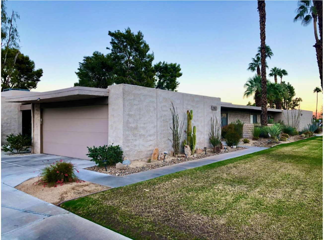
Wexler specified evenly spaced decorative screeds, or vertical lines, for larger expanses of the troweled stucco, as seen here along E. Sandalwood Drive. This subtle element adds interest while remaining modern and minimal. (Photo by Claude Peck)
