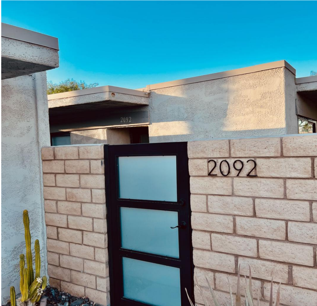
The replacement gate at this two-bedroom unit is one that has been used by other owners, with approval of the Sagewood Architectural Committee and Board. Guidelines ask that gates be simple, unadorned and of the same height as the adjacent block walls. The simple, sans serif address numbers are in keeping with a desire to have those be consistent throughout the complex over time. (Photo by Claude Peck)
