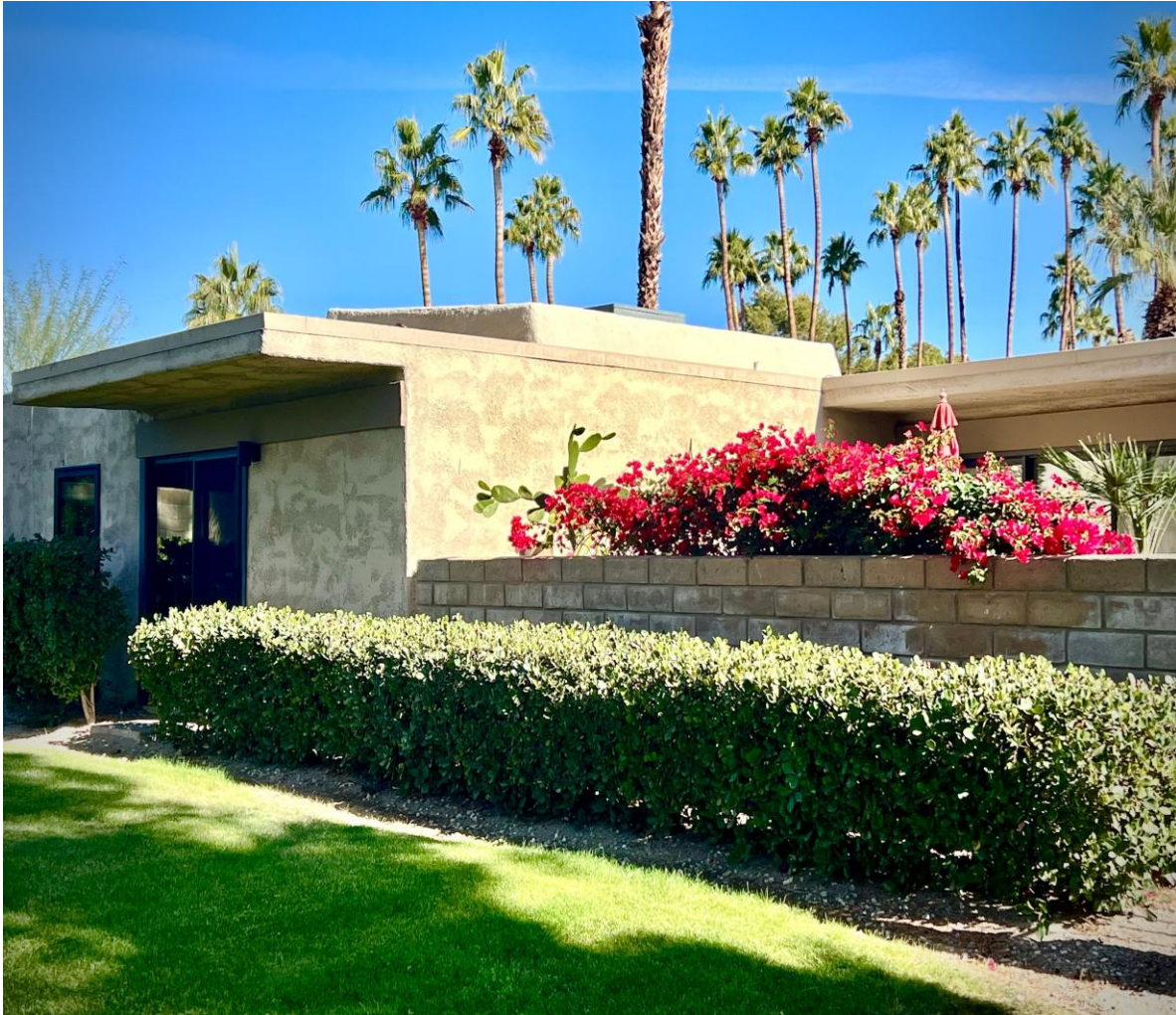
Character-defining features of Donald Wexler's Sagewood include right angles, play of sunlight and shadow, cantilevered roof extensions, slumpstone enclosures for private patios, and orientation to shared green spaces. (Photo by Claude Peck)
